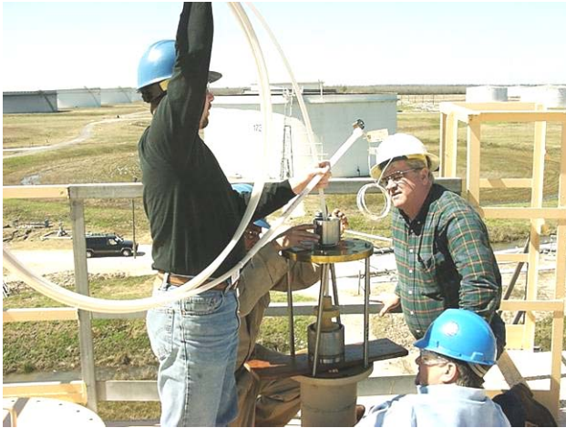
Installing Flexible DataStik ™ (for tanks up to 50 ft.)
